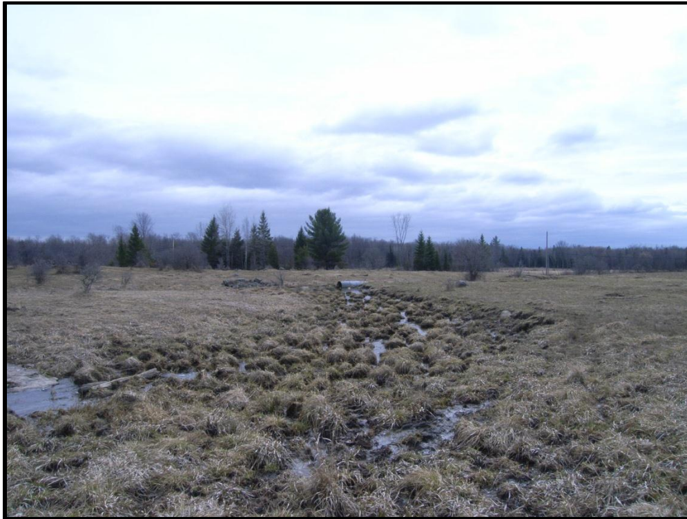
Photograph 46. Ill-defined and highly degraded reach of Monck Road drainage feature 2 with exposed culvert.
